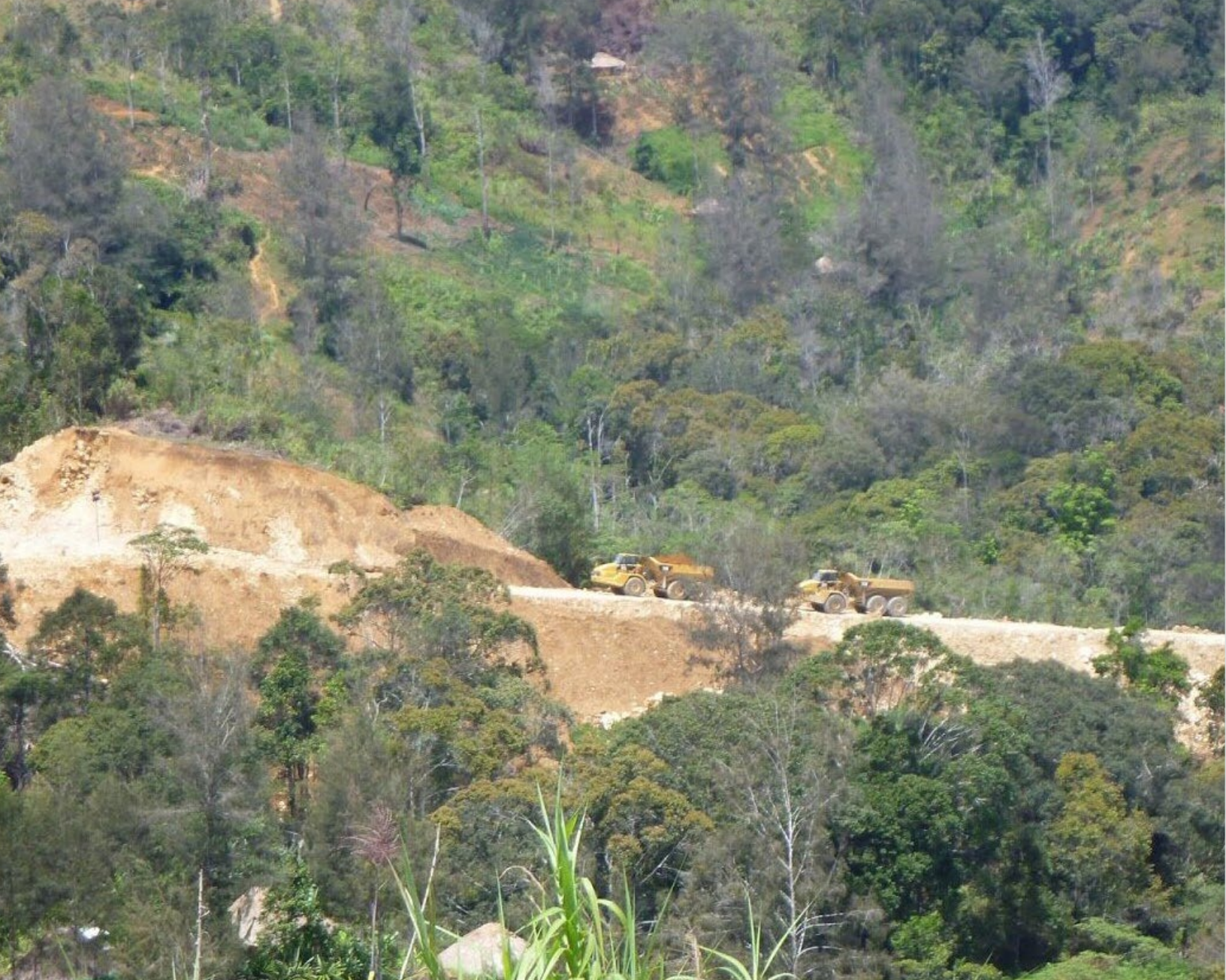
PNG LNG construction phase © James McIlraith / University of Otago
